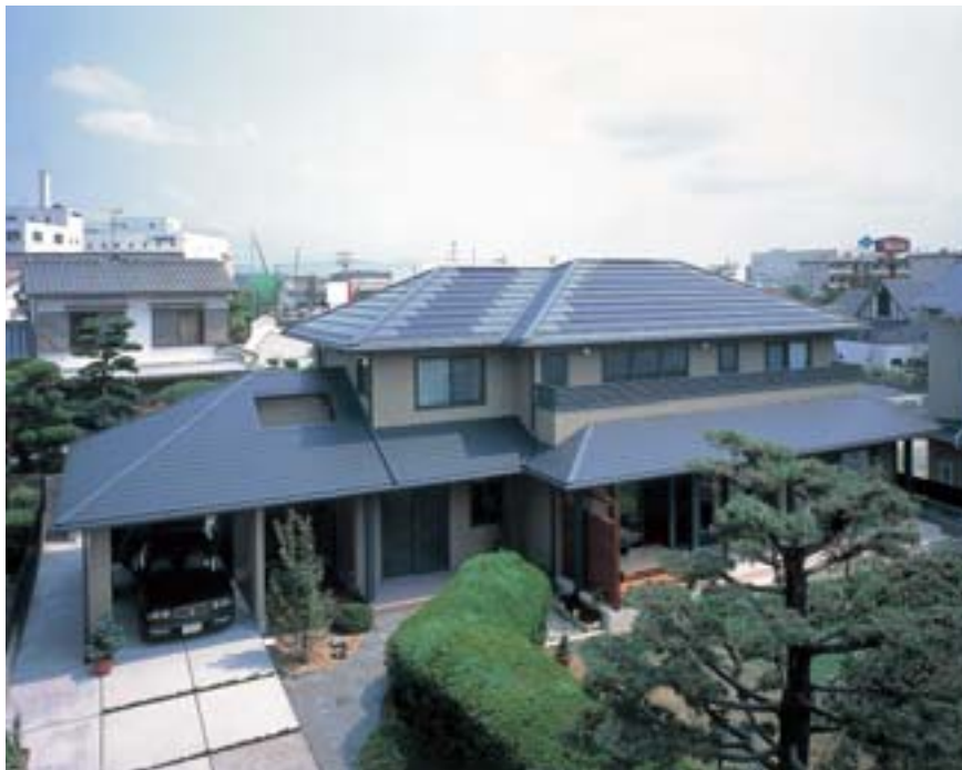
Photovoltaic for a house
