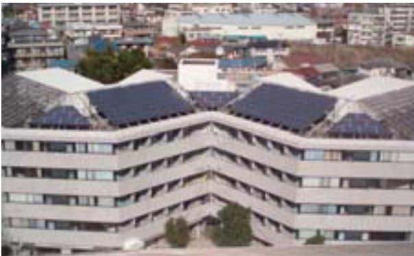
Apartment house (installed capacity: 20 kW) New College Town Management Association Corporation (Tokyo)
