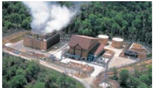
Tohoku-Electric Power Co., Inc. Sumikawa Geothermal Power Plant (50MW)
