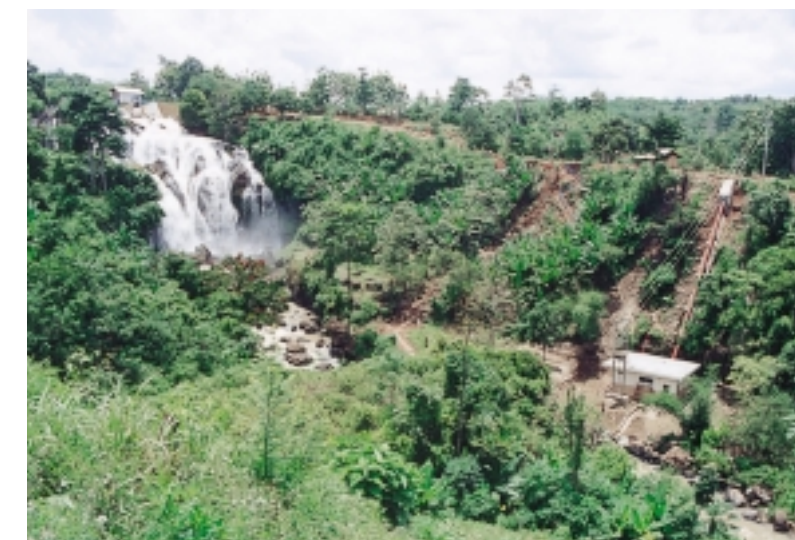
Dispersed small scale hydroelectric power plant (Indonesia)
