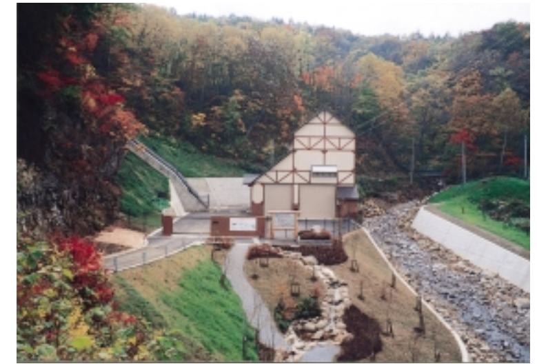
Iwate Prefecture Matsukawa Power Plant (4,600 kW)
