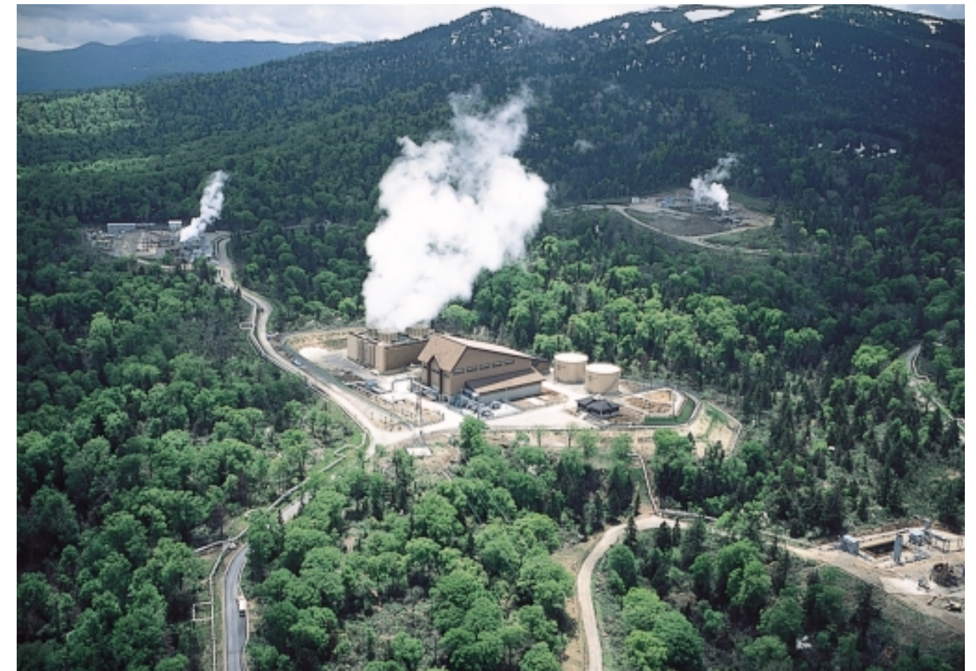
Sumikawa Geothermal Power Plant (capacity 50 MW), Tohoku Electric Power Co., Inc.
