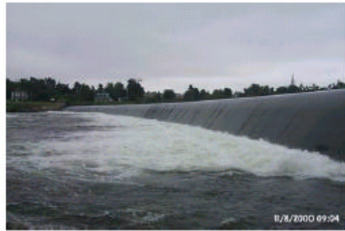
Chambly Dam on the Richelieu River
