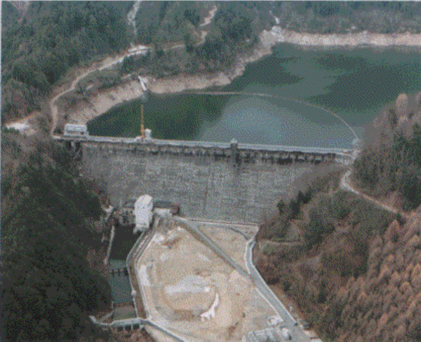
Miura Dam (Miura Power Plant) Maximum output : 7,700kW Maximum discharge : 17.5m 3 /s Effective head : 54.7m
