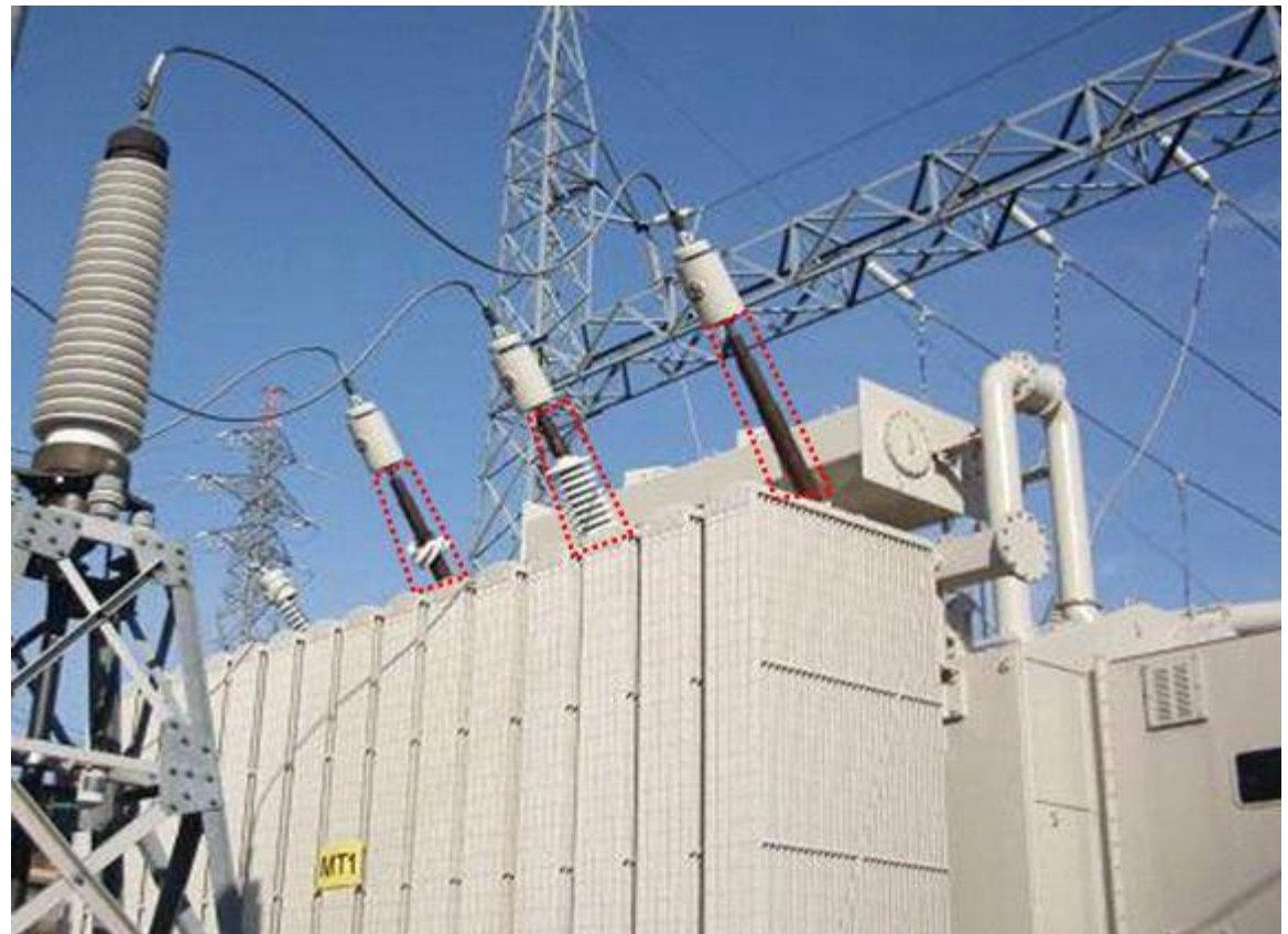
Damaged transformer bushing
