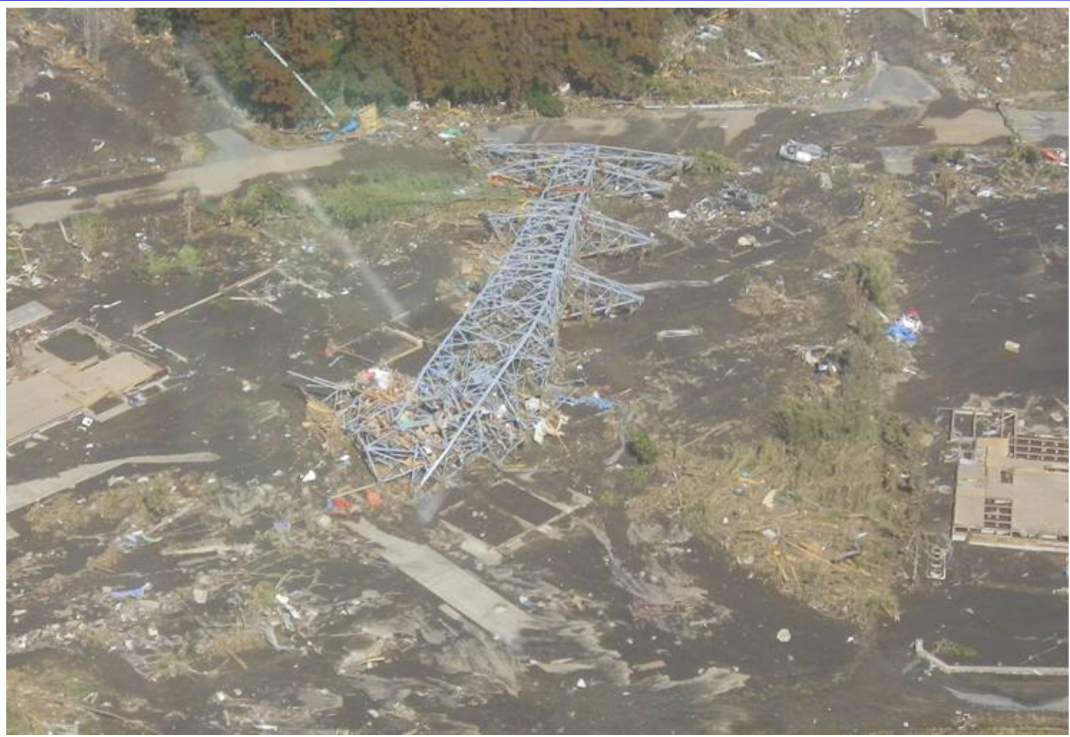
Tsunami damage (Collapsed steel tower)
