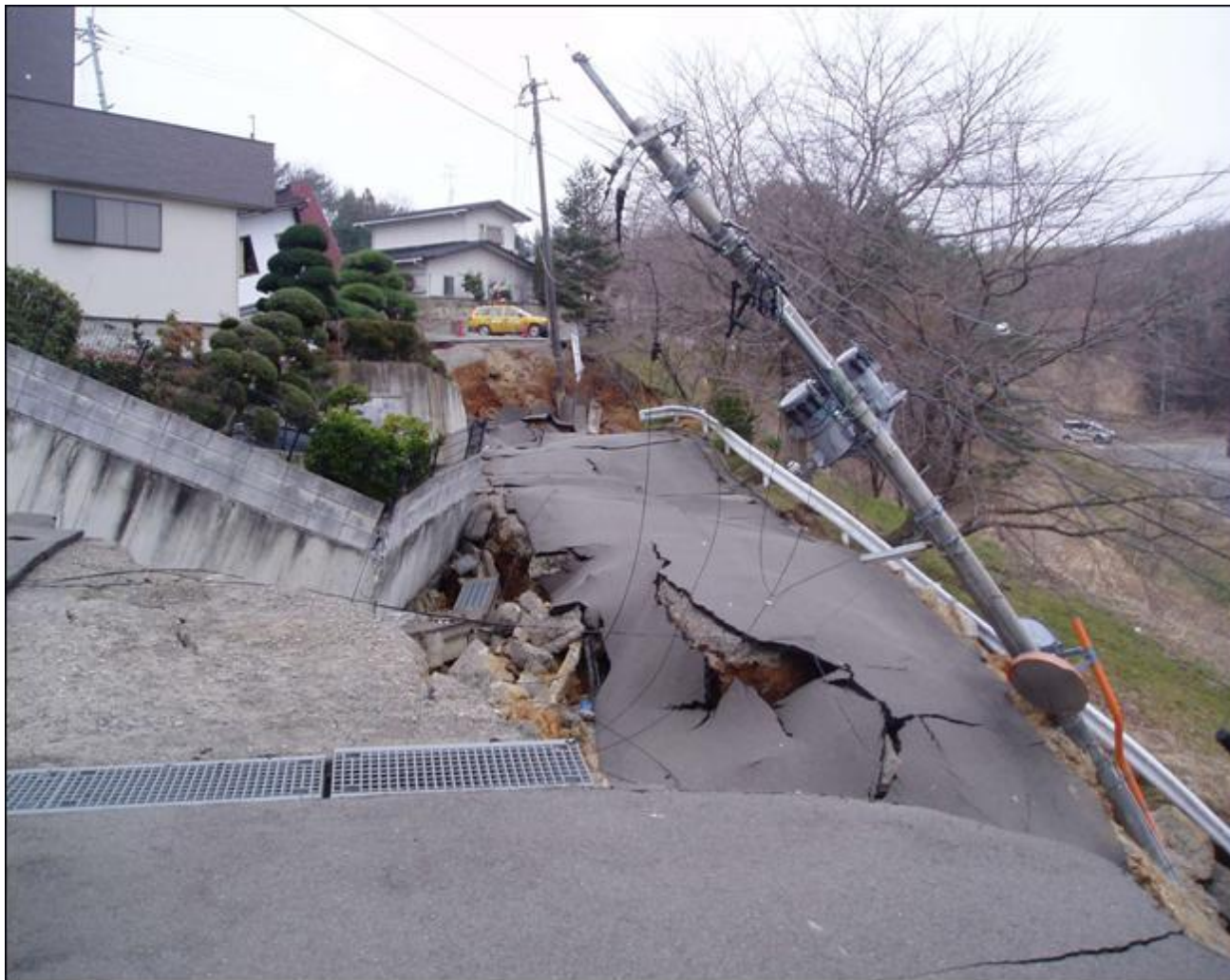
Pole inclined due to damage to the road (Fukushima City, Fukushima Prefecture)
