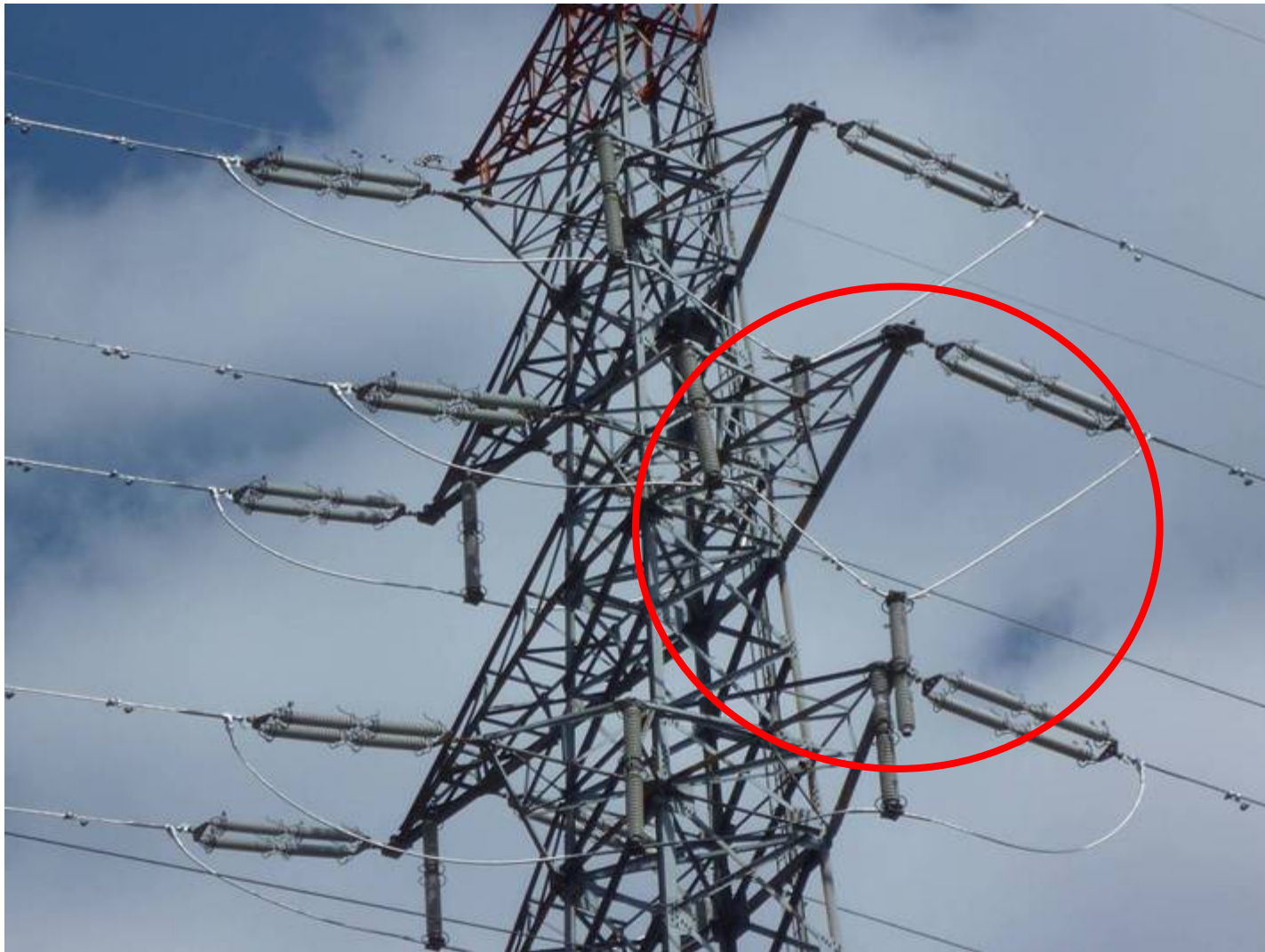
Broken supporting insulator
