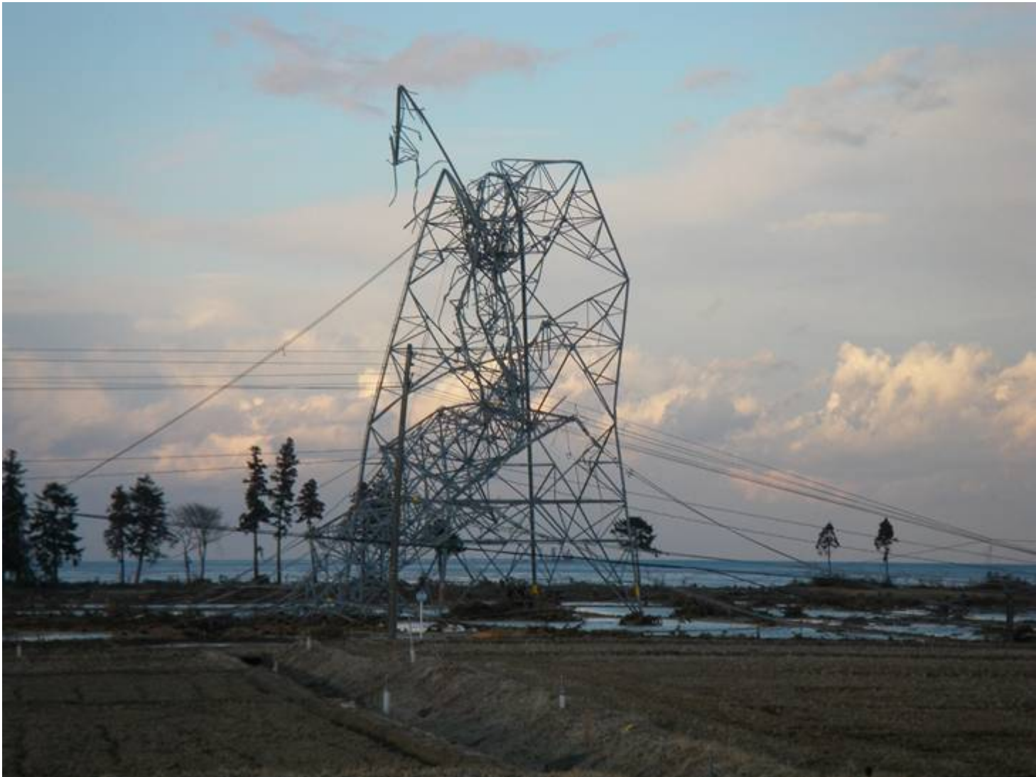
Tsunami damage (Broken steel tower)
