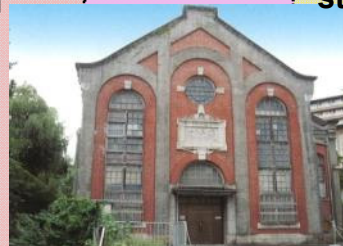
Power house at 2nd stage (existing)
