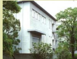
Power house at 3rd stage (in-service)
