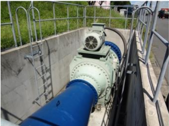
Siphon type Intake System for turbine installed on Discharge Drain
