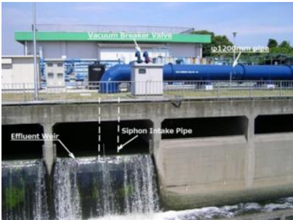
Siphon type Intake System for turbine installed on Discharge Drain
