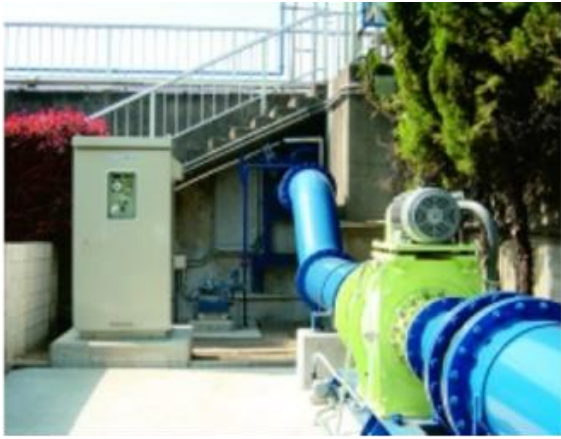
Siphon type Intake System for turbine installed on Discharge Drain
