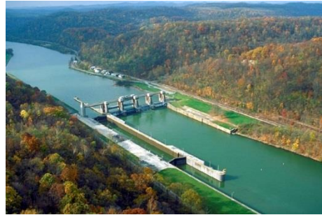
Non-Powered Dams and Conduits
