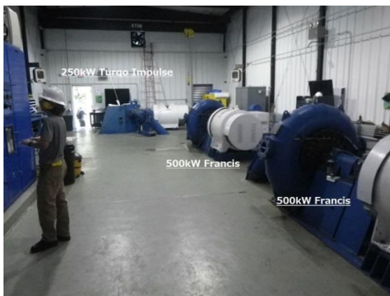
Turbine in Humpback Hydropower House
