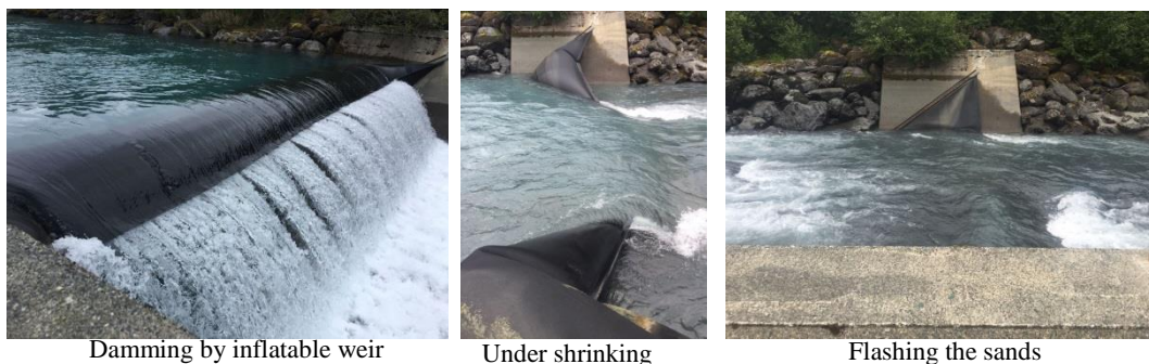
Photo-4 Sand sedimentation flushing by inflatable weir
