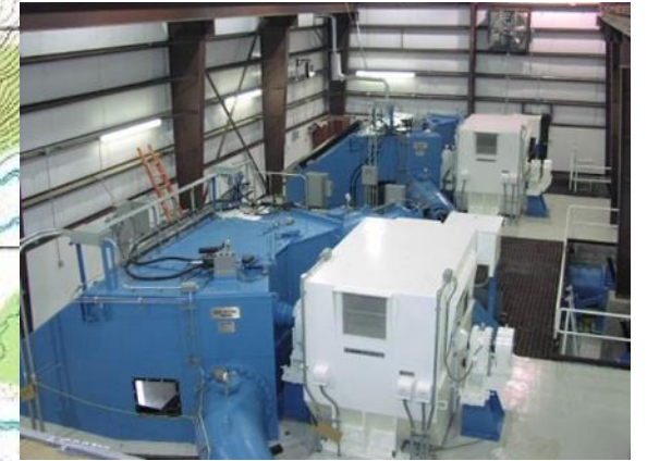
Turbine Generator in Power Creek Hydropower House
