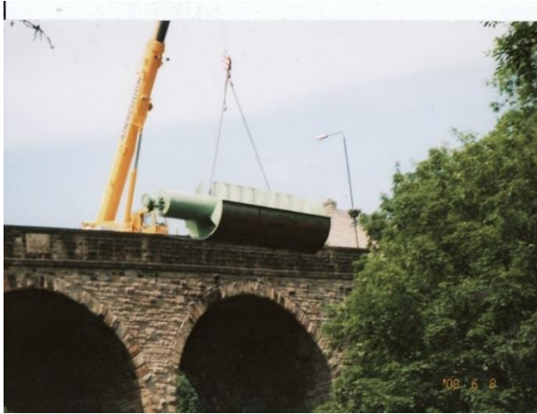
Photo-2 Lowering the turbine from historical Union Bridge [2]
