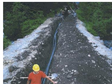
Embedded Transmission line in the trench
