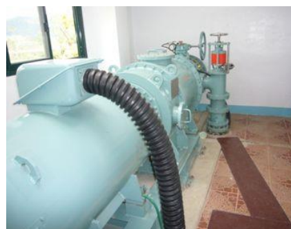
Photo-7: Water turbine and generator
