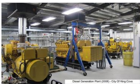
Photo-2 Diesel Engine Generator Units [3]
