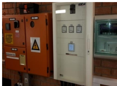
Photo-3 Generator control panel
