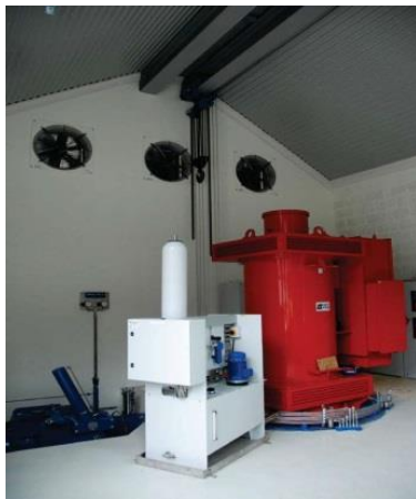
Photo-6 Generator (back) and hydraulic system (front)
