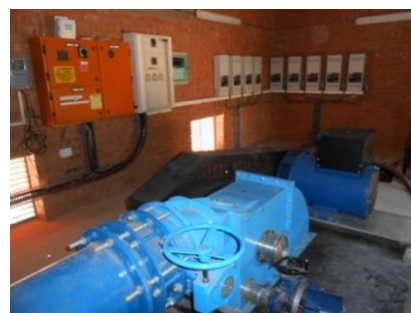
Photo-2 Turbine, generator
