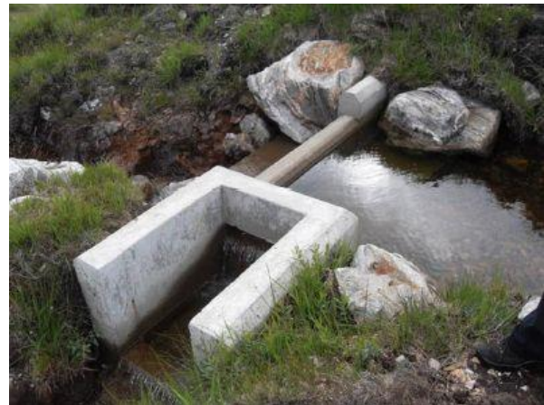
Photo-2 Secondary Intake
