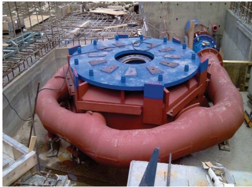
Photo-4 Turbine casing (under construction)
