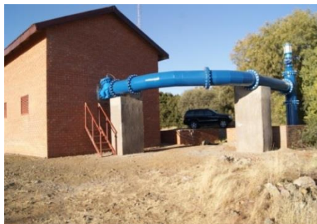
Photo-1 Penstock and powerhouse
