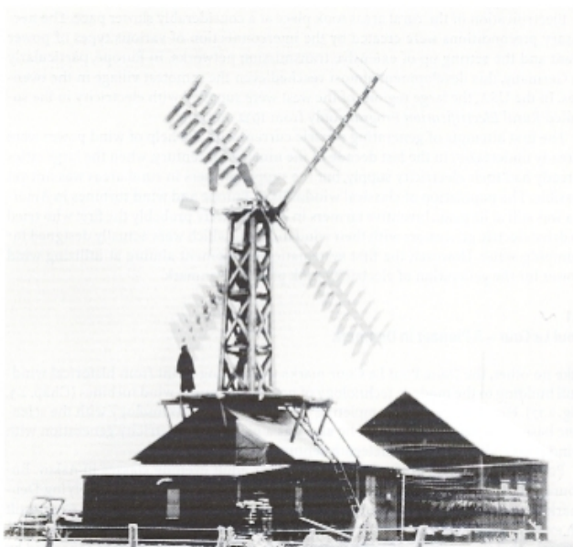
Fig. 2.1. Poul La Cour's first electricity producing wind turbine in 1891 in Askov, Denmark [1]
